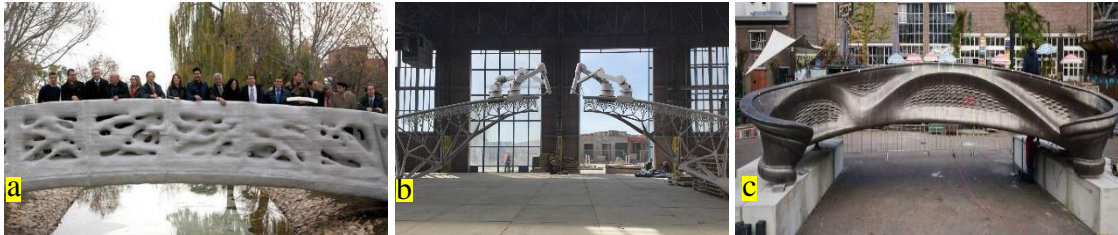
Fig. (2) (a) 3D printed bridge with the D-Shape technology. The first structure of this type in the world [7] , (b) 3D-printed steel bridge in the heart of Amsterdam 3D-printed steel bridge in the heart of Amsterdam, (c) the first 3D-printed steel bridge. In 2015, Dutch 3D printing company MX3D [8] .
